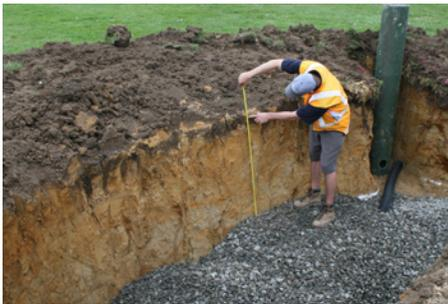
Fig.2 Checking level of gravel bedding with overflow runoff riser and underdrain and connection slot in place.
