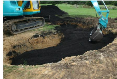
Fig.3 Soil mix placed to compact naturally.
