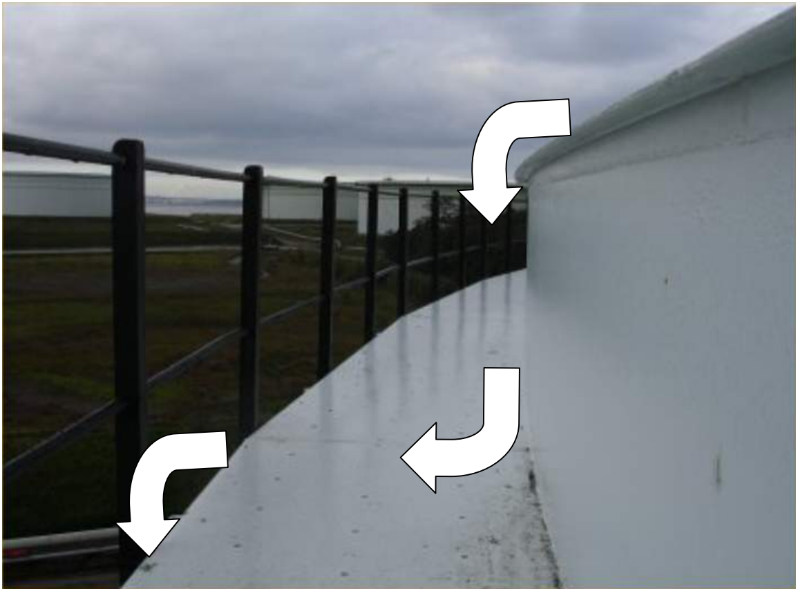
Figure 4: Windgirder/walkway at the top of a typical floating roof tank. The arrows indicate liquid path in the event of overfill.
