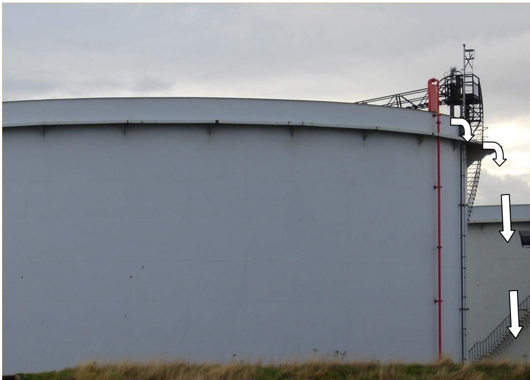
Figure 5: Wide view of windgirder/walkway at the top of a typical floating roof tank. The arrows indicate liquid path in the event of overfill
