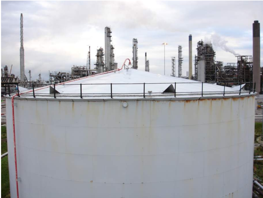
Figure 1: Typical (Buncefield type) petrol tank – shrouded vents around the tank perimeter
