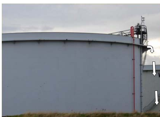
Figure A2: Windgirder/walkway at the top of a typical floating roof tank. The arrows indicate liquid path in the event of overfill.
